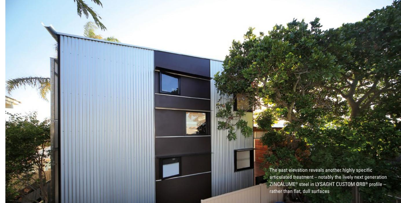
The east elevation reveals another highly specific articulated treatment – notably the lively next generation ZINCALUME® steel in LYSAGHT CUSTOM ORB® profile – rather than flat, dull surfaces
