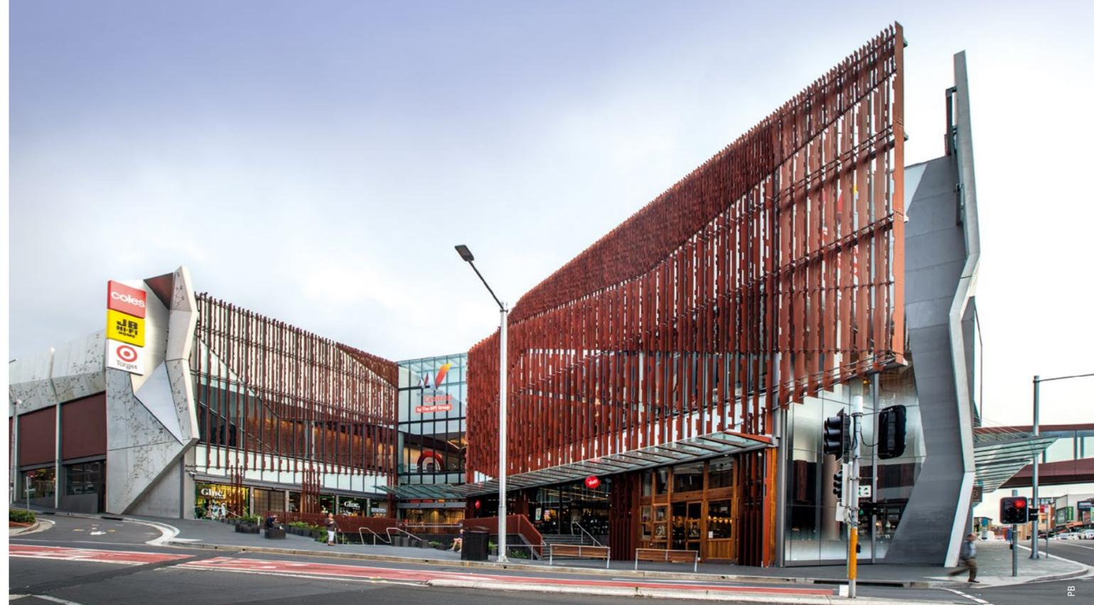
ABOVE: The visual rhythm of the steel blades draws the eye into the south-facing entrance of the building, which is located on a significant gateway site in Wollongong's CBD
