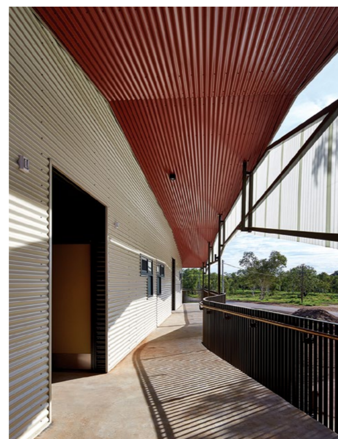
ABOVE: The verandahs, circulation spaces and outdoor common areas are shaded using timber slats and polycarbonate screens mounted on steel frames, which create abstract patterns that reference local artworks
