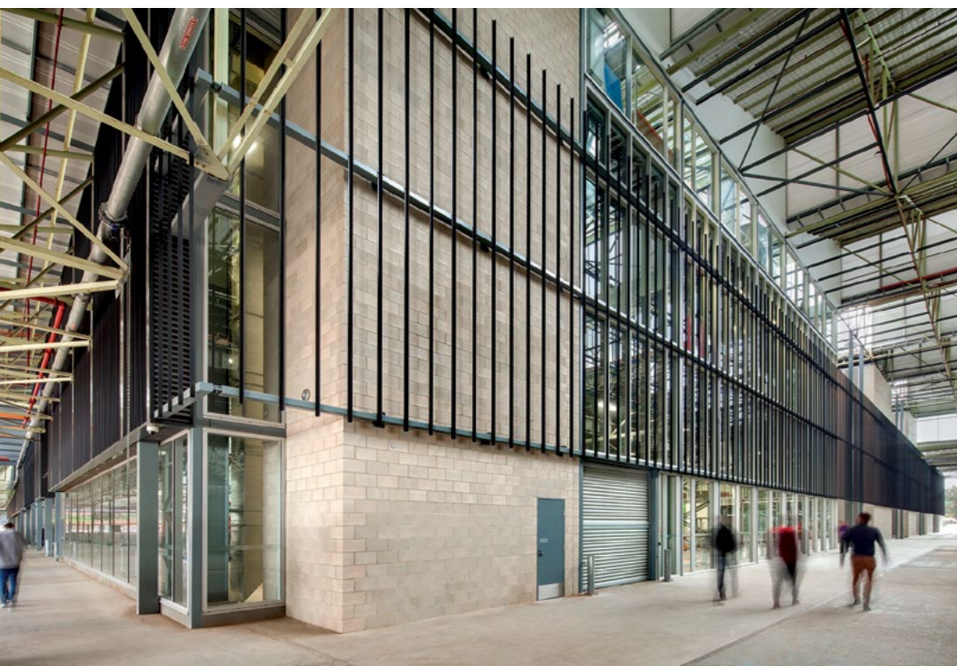
The rigid geometry of the original structure, and its different roof heights ranging from six to 15 metres, dictated the dimensions and placement of the new workshops (top), teaching spaces and offices (bottom left), and main circulation spaces (bottom right) within the existing envelope
