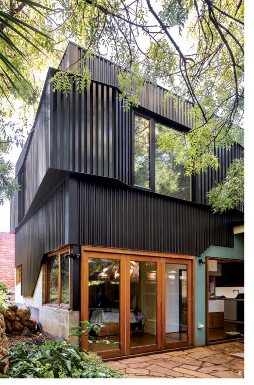
LEFT AND BELOW: COLORBOND® steel in Stramit Longspan® profile, in the colour Nightsky®, wraps sympathetically around the existing timber and concrete-block envelope
