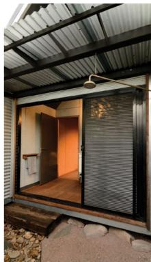
The steeply pitched roofs help to disperse torrential rain from tropical downpours quickly, and the quirky gutter detail was worked out on site, after mis-measured roof sheets were delivered
