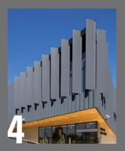
Bamford-Architects creates a bold civic gesture for a new Melbourne police station by handsomely wrapping it in custom-folded COLORBOND® steel cladding
